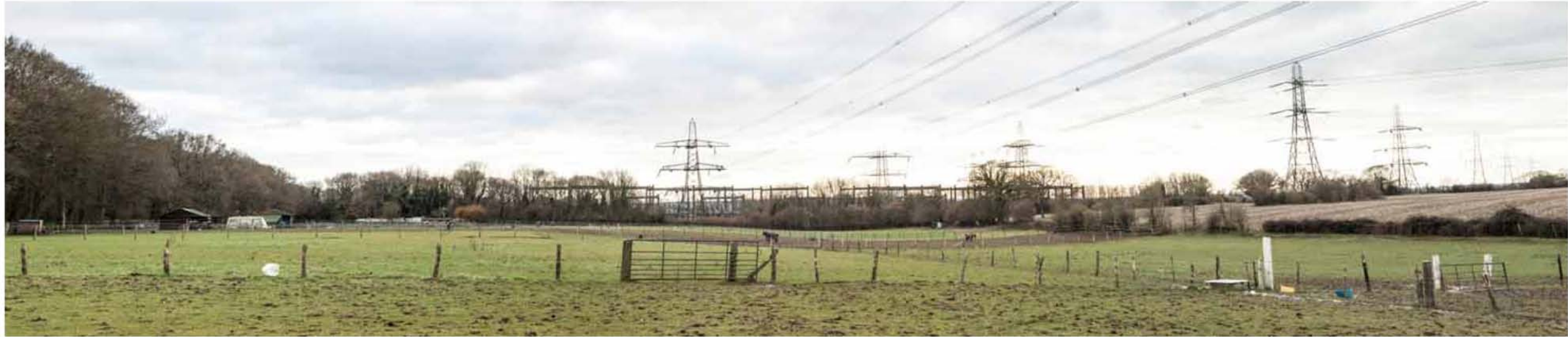
View 1 towards the substation, existing situation, winter 2012/2013.
