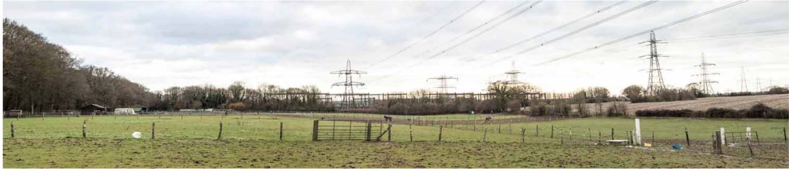
View 1 towards the substation, existing situation, winter 2012/2013.
