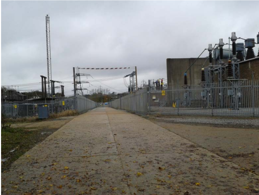
Photograph 3 – Site compound entrance 1
