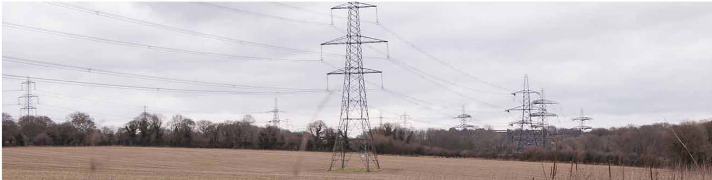
View 4a of the existing situation, towards Lovedean Substation and proposed extension (Winter 2012/2013).
