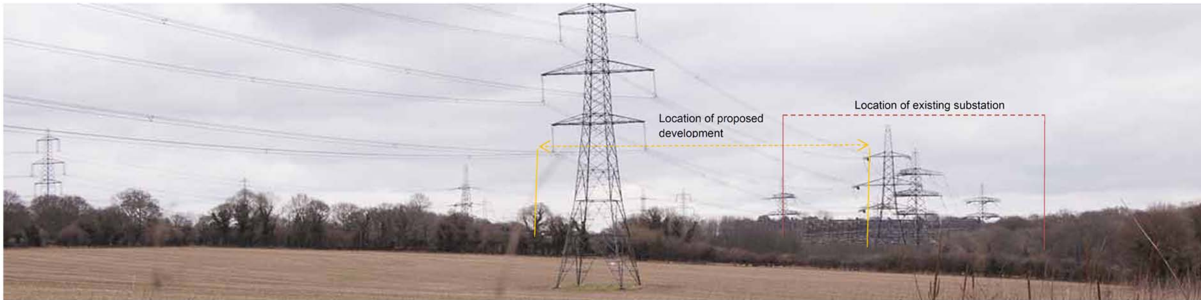
View 4a year 1, towards Lovedean Substation and proposed extension (winter view). The 21m high existing substation gantries and electrical equipment are more visible because of the proposed western boundary tree felling. The 13m tall shunt reactor 7 installation is relatively inconspicuous in comparison with the existing substation to the rear. The proposed feathered trees and extra heavy standard trees would partially screen the lower part of the proposed development and existing substation.
