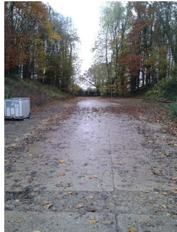
Photograph 2 – Site access road.
