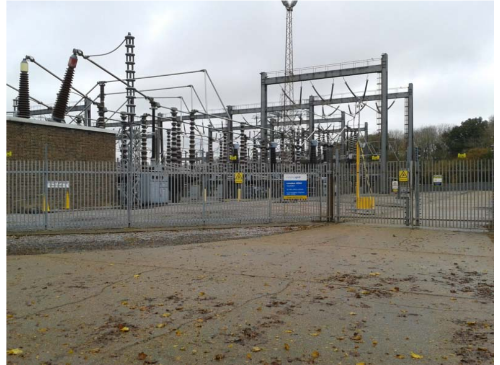
Photograph 4 – Site compound entrance 2
