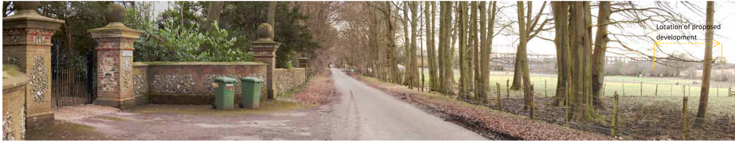
View 1b of the existing situation towards Lovedean Substation and proposed extension, viewed from entrance to Hinton Daubney on Broadway Lane at the edge of the South Downs National Park (winter view). The proposed development would be visually imperceptible, screened by a combination of landform, the existing substation and distant trees.
